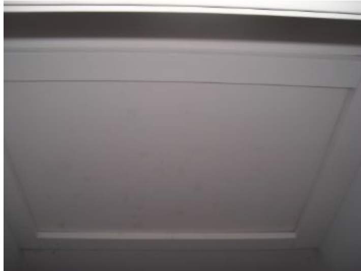
access in upstairs bedroom closet.
